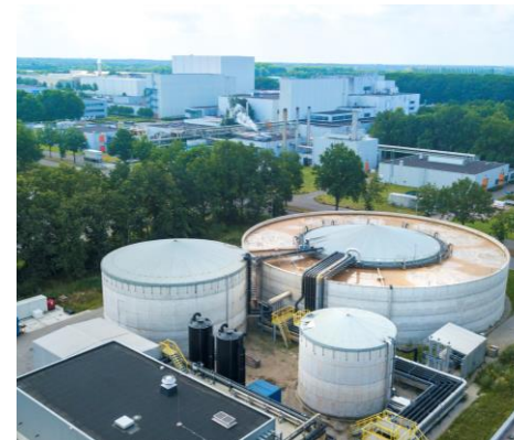
On-site waste water purification
